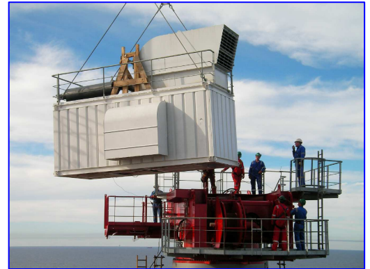
Lifting Of Crane Machinery House
