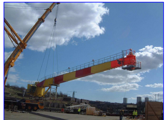
Lifting Of Crane During Load-out
