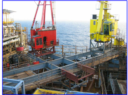
Crane Replacement Using Modular Skidding
