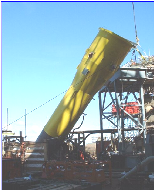
Offshore Pedestal Replacement
