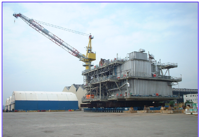
New Build Crane Pre-Installed on New Offshore Module
